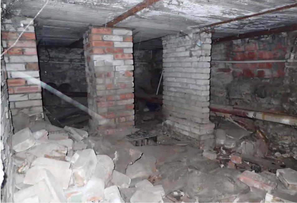
A photograph showing the interior of a severely damaged room. The walls are made of brick and are crumbling. Two prominent brick pillars support the ceiling. The floor is covered in a large amount of rubble, including broken bricks, concrete, and debris. A white pipe runs diagonally across the room. The lighting is dim, highlighting the extent of the destruction. |
