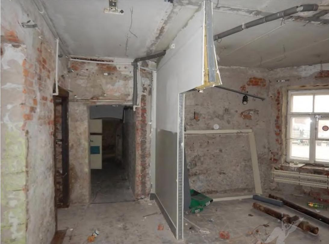
A photograph showing a room where a partition wall is being demolished. The wall is partially removed, revealing the brick structure underneath. Debris, including pieces of wood and plaster, is scattered on the floor. A window is visible on the right side. The ceiling has exposed pipes and some structural elements.       |
